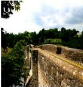
Teaton Bridge from south
